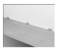
Place a row of full-size 4 mm panels (clear adhesive downwards) overlapping the second row of the 3 mm panels halfway.
