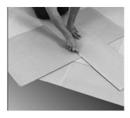
Maintain a gap of at least 6 mm between panels and walls. Start at the shorter wall of the room with a row of 3 mm panels cut in half lengthways (coloured adhesive uppermost).
