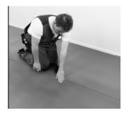
Forbo QuickFit can be cut from the top using a straight cutting blade, and then snapped.
