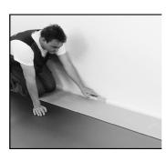
Place a row of full-size 3 mm panels (coloured adhesive uppermost) staggered against the first row of the cut the panels - ideally in a brick design as shown above.
